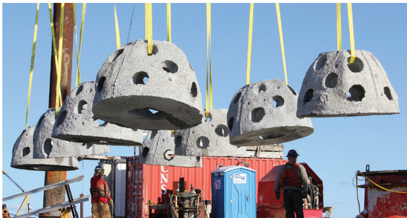
Placing reef balls at Sabin Point in Riverside, Rhode Island.
