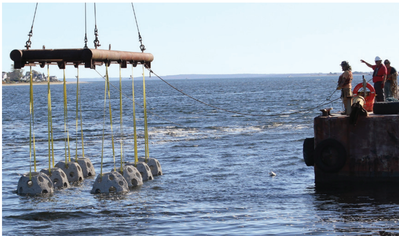
Placing reef balls at Sabin Point in Riverside, Rhode Island.
