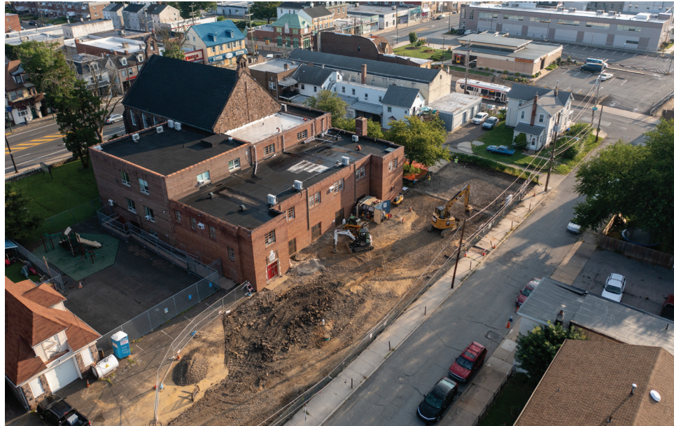
A drone captures construction activities at the Holmesburg Baptist Church and Christian Academy in Northeast Philadelphia, where TNC is working with the landowner on a series of new green stormwater infrastructure projects. © Oak Leaf Media
