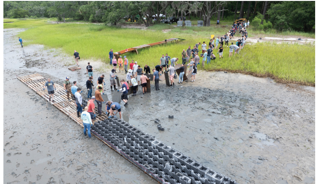
TOP TO BOTTOM: A construction team installs wooden breakwater poles at the Boyd Living Shoreline. © Tanya Ackerman; Marine and civilian volunteers stack Oyster Castles™ to build a reef at Marine Corps Air Station Beaufort. © Paul Nurnberg
