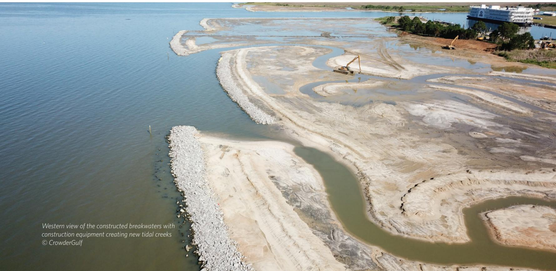
Western view of the constructed breakwaters with construction equipment creating new tidal creeks © CrowderGulf
