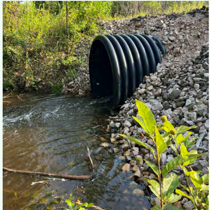
Culvert in stream crossing in East Texas. © TIG and subsidiaries
