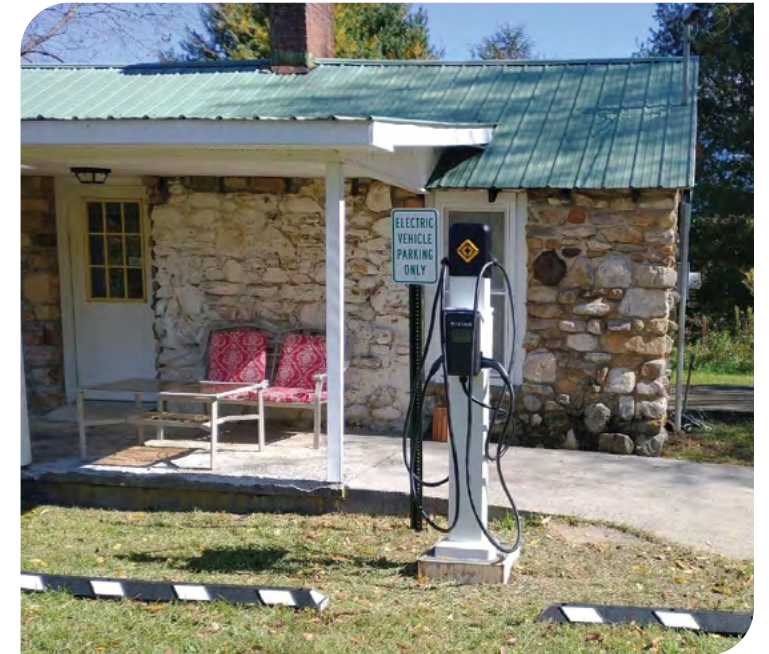
Rivian EV Charging Station at the Orchard Bog Preserve © TNC
