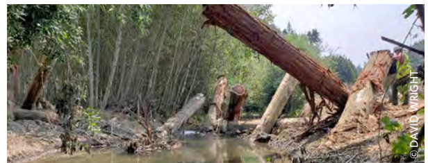
AN ENGINEERED LOG JAM THAT TNC CREATED FOR SALMON HABITAT ON TEN MILE RIVER.
