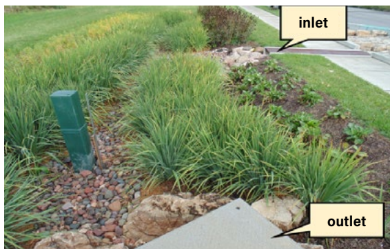
Figure D4.1 | A bioretention system designed to treat nonpoint source runoff from an urban landscape
